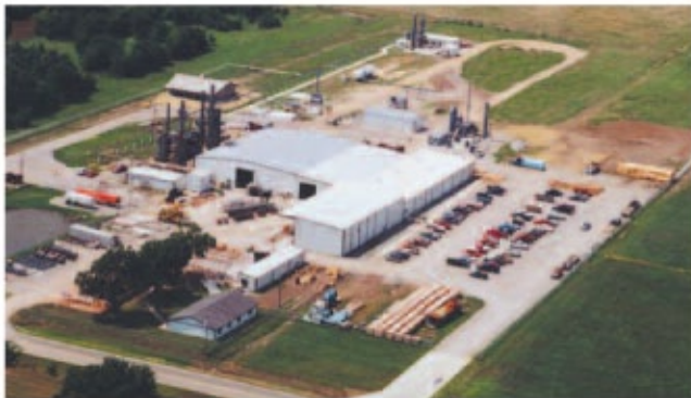
Callidus research, development and manufacturing facility
